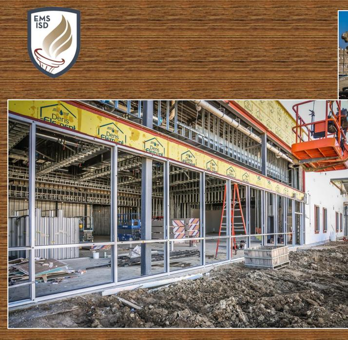
Storefront frames have been installed in the cafeteria. Landscaping, trenching, and main lines are being installed.
