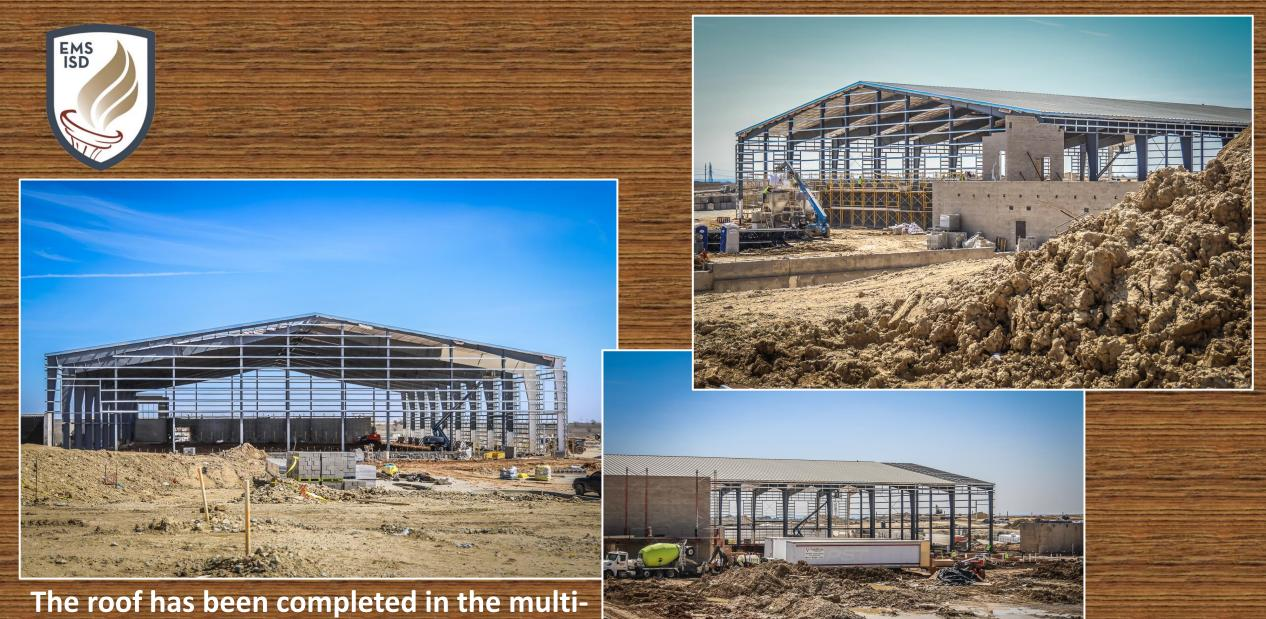
The roof has been completed in the multipurpose building. CMU block has begun on the walls.
