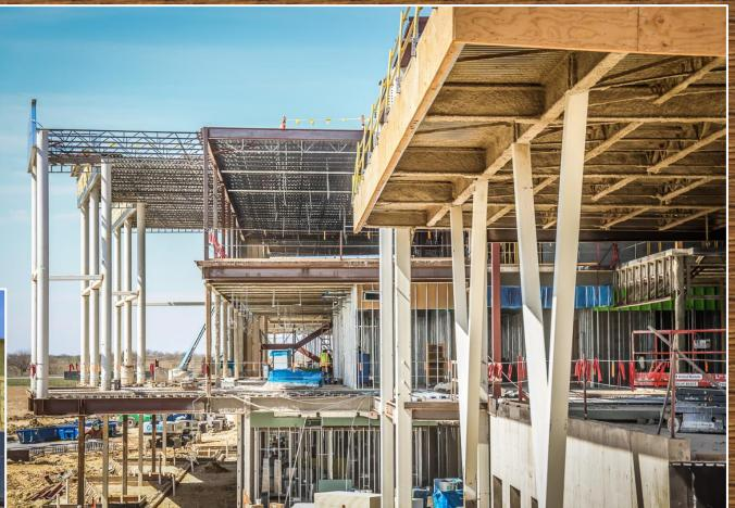
Interior metal studs continue to be installed along with rough-in mechanical and roofing on the main academic building.
